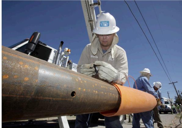
TEP uses greater mil thickness than the industry designed standards on the embedded portion of the pole, taking special care to understand the geotechnical aspects of the soils in order to avoid corrosion over the lifetime of the pole.
